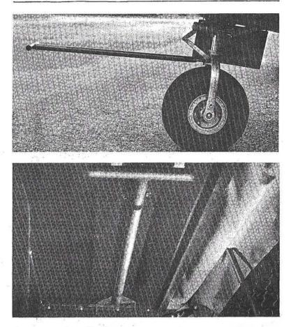
held in position by its connections with the steerable nosewheel and does not need to be secured except under unusually high wind conditions. The flaps are locked in position when left full up, so should always be retracted for mooring to prevent wind damage and permit using the flap as a step.
